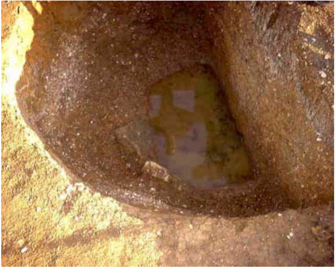
A fine example of a quarried pit where the pea-gravel has been removed and a water store has been built in-situ. Note the stone faced sides to the water store backed by non-porous clay.
