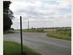
The Give Way sign on Mill Road is missing
