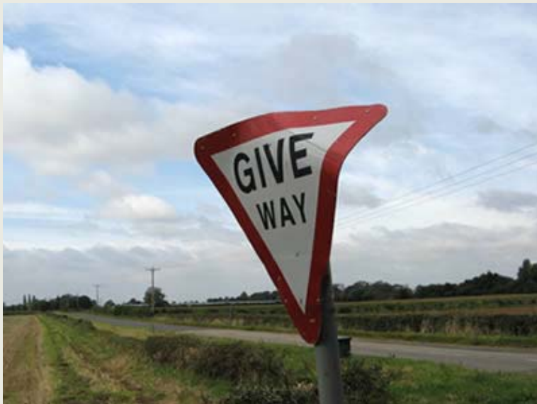
One that got away - for now. The Give Way sign at the Maxey Road / Mill Road crossroads beside the church shows evidence of damage due to attempted forced removal.
